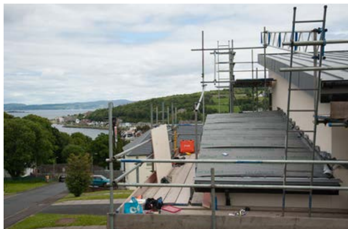
From beach views to building upgrades, retrofit works progress on WHHA homes in the heart of the Isle of Tiree community.
